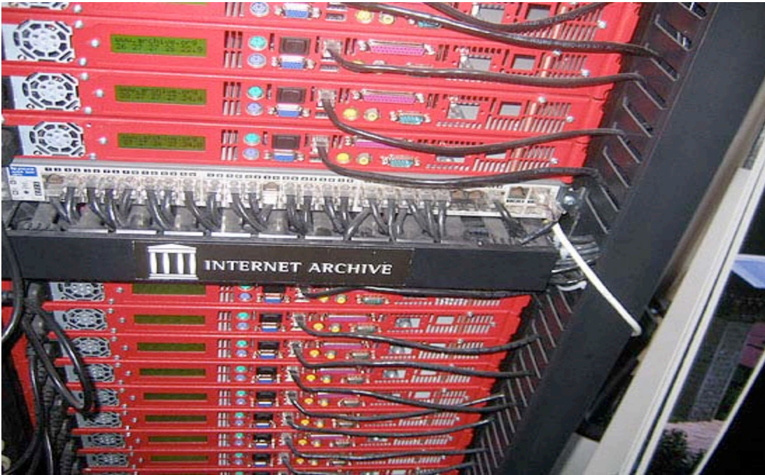
Figure 27. "The bits go here. A sample Internet Archive server rack, encompassing a petabyte of storage. A petabyte is 1000 terabytes, and a terabyte is 1000 gigabytes," Kirschenbaum 2007; Petabox 2009
